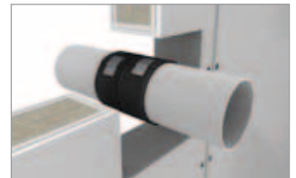
Fixing of the finished wrappings with duct tape
