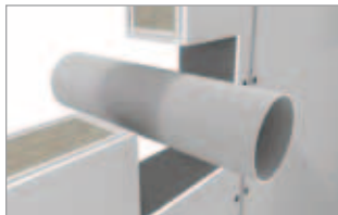
Clean reveals and rough opening
