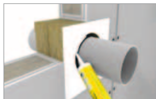
Sealing of the ring gap with HENSOMASTIK® 5 KS SP
