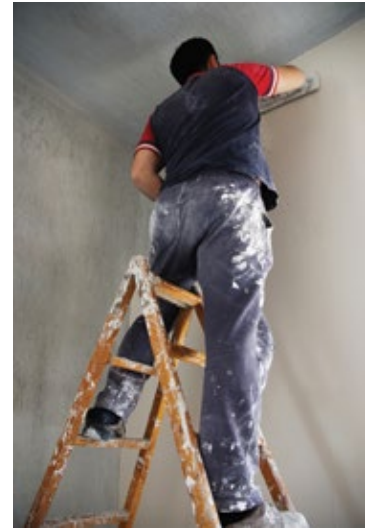
Plastering the board joints in partitions (above left) and the junctions of wall and ceiling (above right)
