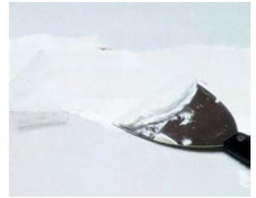
Applying joint filler
