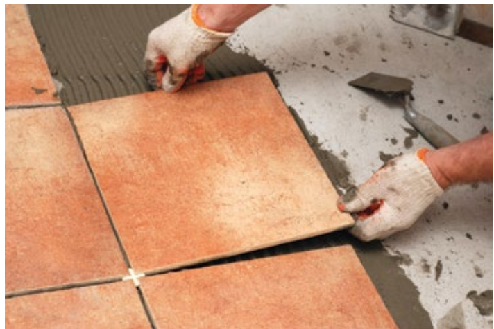
Applying tile adhesive on pre installed Promat boards prior to tiling
