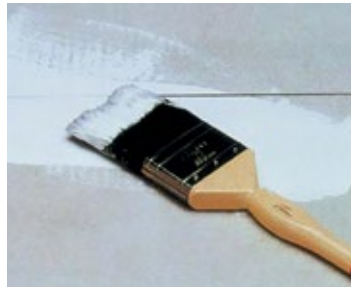
Preparing joint with primer
