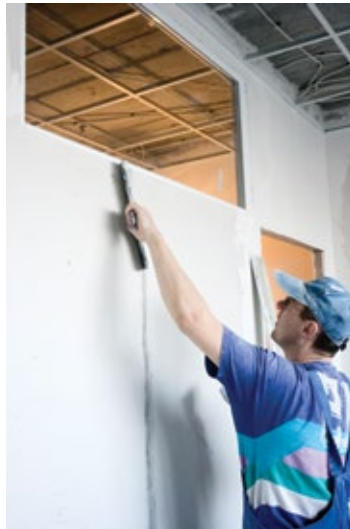
Plastering the board joints in partitions (above left) and the junctions of wall and ceiling (above right)
