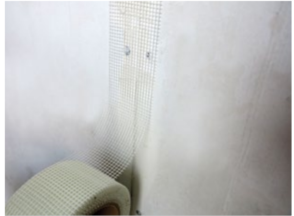
Fill joint with single, thin layer of plaster and then overlay reinforcing mesh
