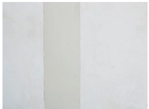
Final joint after finishing with trowel
